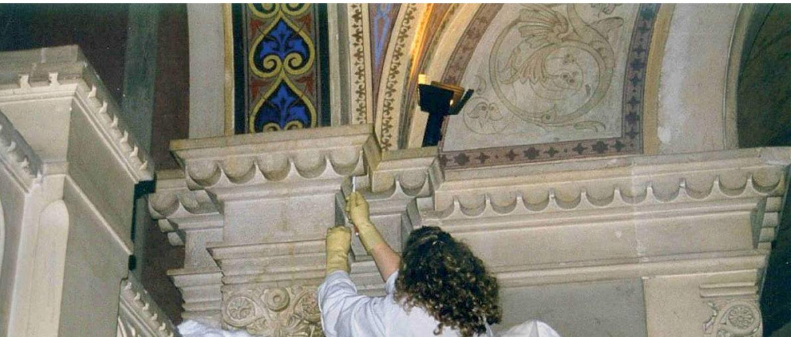
Fig. 4 Cleaning phase on the stucco elements.
