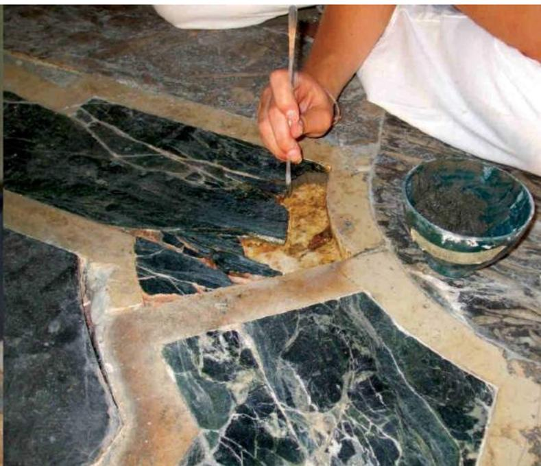
Fig. 32 (left) Retouching by dots on the biggest losses.
