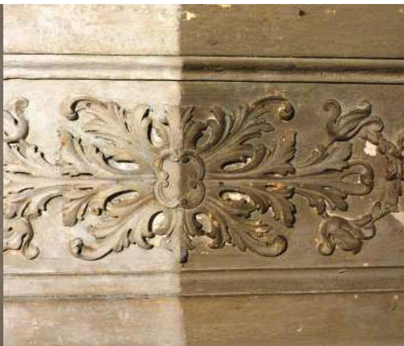
Fig. 47 (left) Cleaning sample performed on the overpainted surface in order to identify the layer to unveil. Fig. 48 (right) Details the reliefs of the gallery during cleaning.
