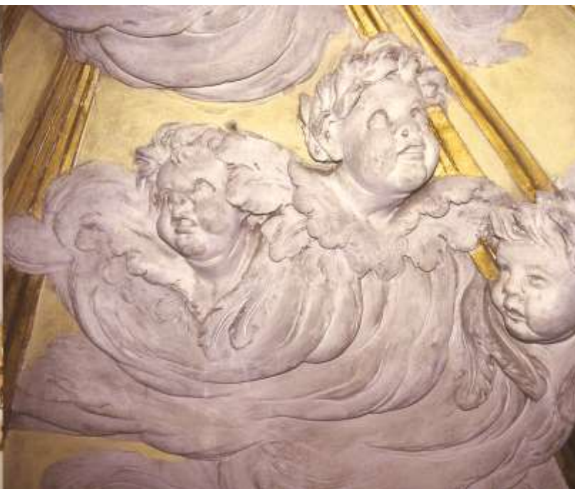
Fig. 60 (left) View of the chancel, after restoration. Fig. 61 (right) The stuccowork above the main altar, before restoration.
