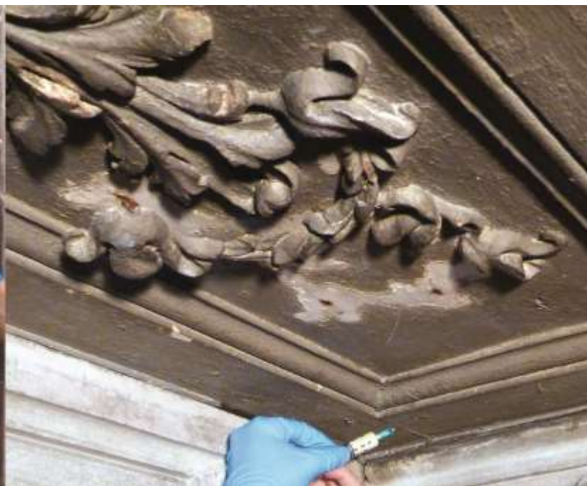
Fig. 45 (left) Consolidation of a disjointed element of the reliefs representing musical instruments in the highest section of the choir balcony.
