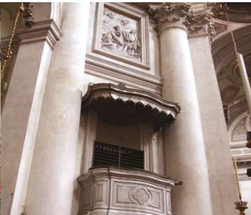
Fig. 41 (left) Chapel of St. Dominic, after restoration.
