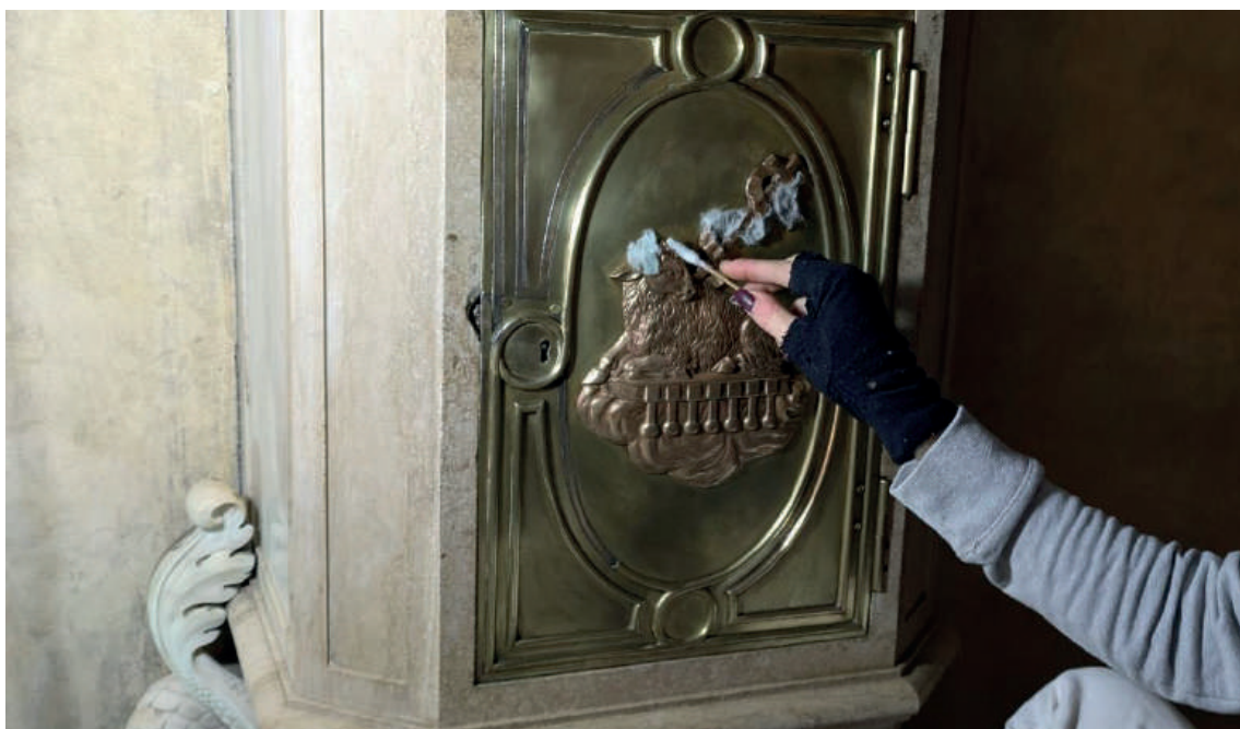
Fig. 35 - Degradation of the stone that composes the baptismal font.
